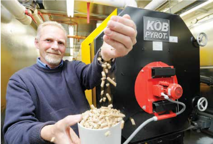
Former UNBC employee Doug Carter shows off the pellets used as fuel in UNBC's wood pellet heating system.
