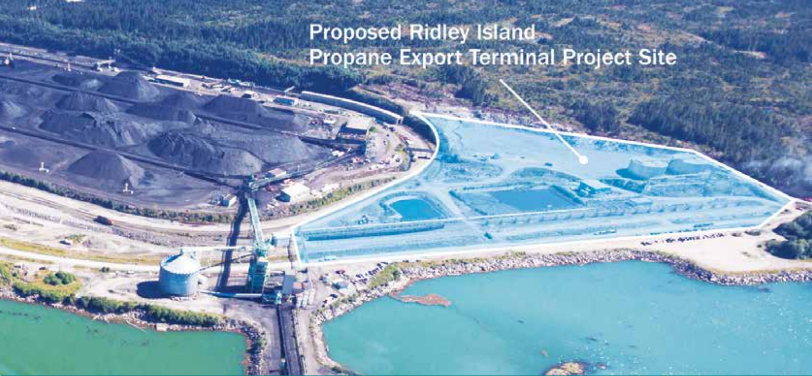
Ridley Island Propane Export Terminal Project site.
