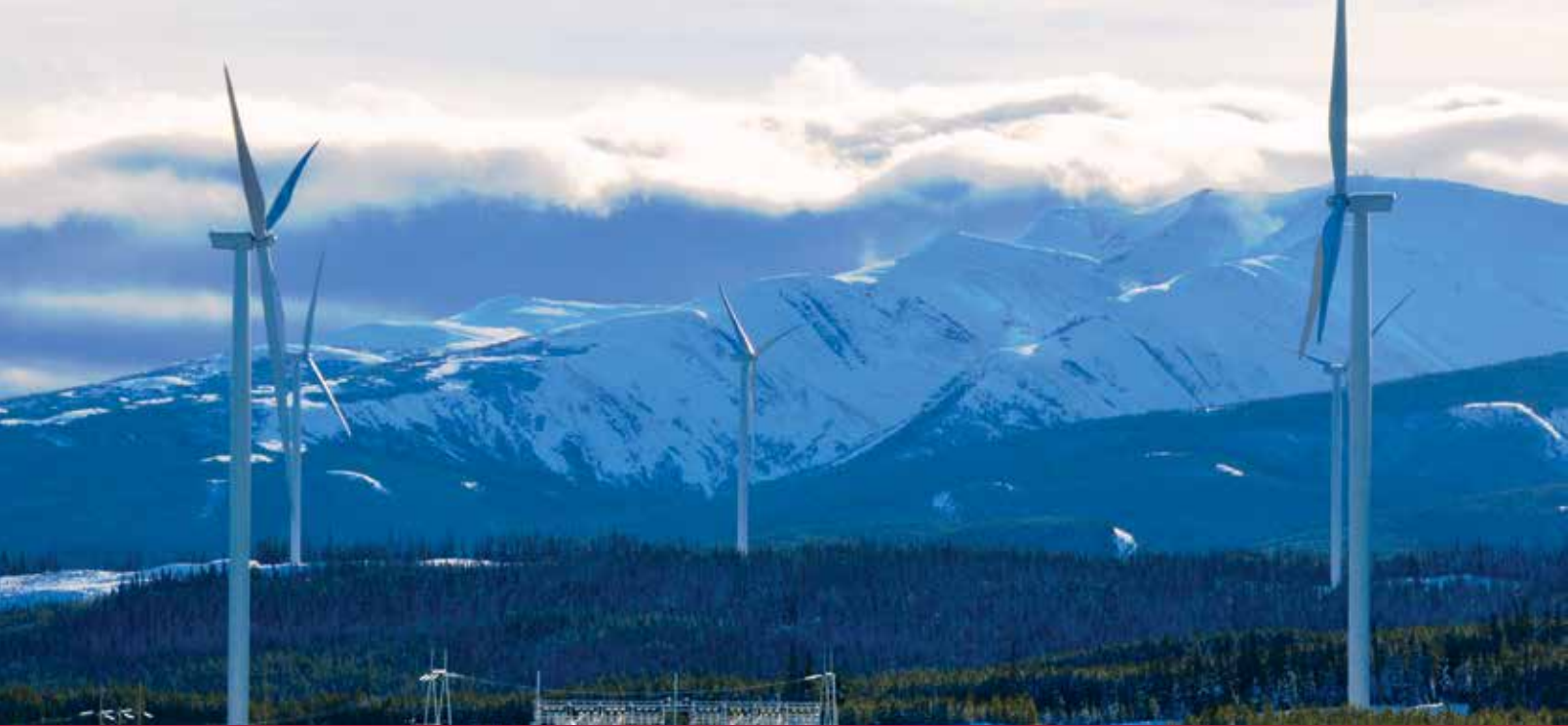
The Meikle Wind Project in Tumbler Ridge, B.C. is the largest wind facility in the province.
