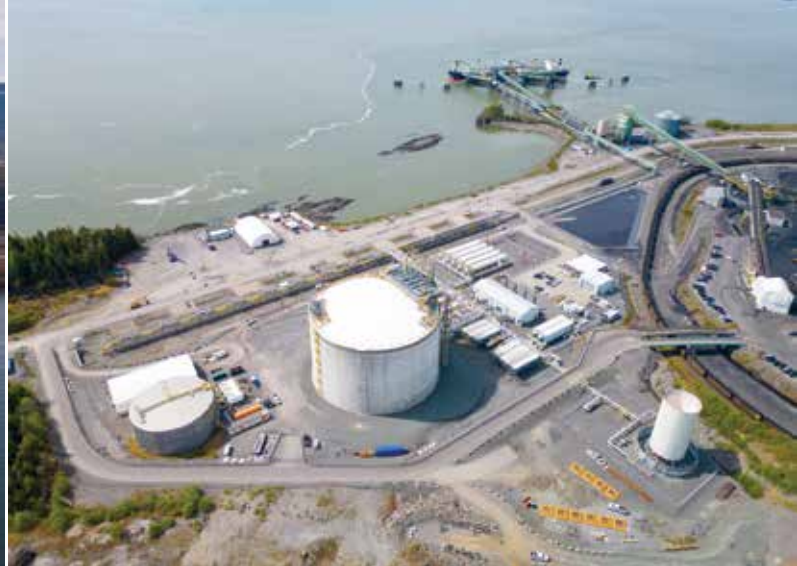
The Ridley Island Propane Export Terminal.
